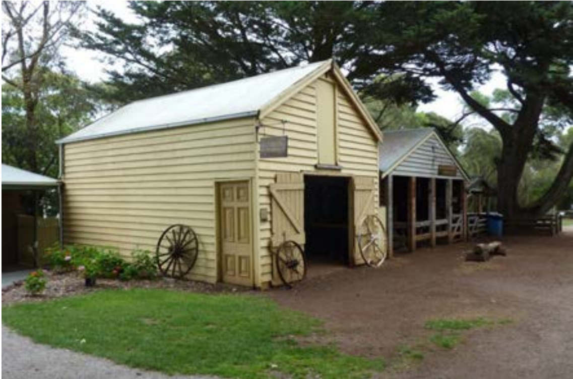
Figure 57 Amess stables looking north-west
