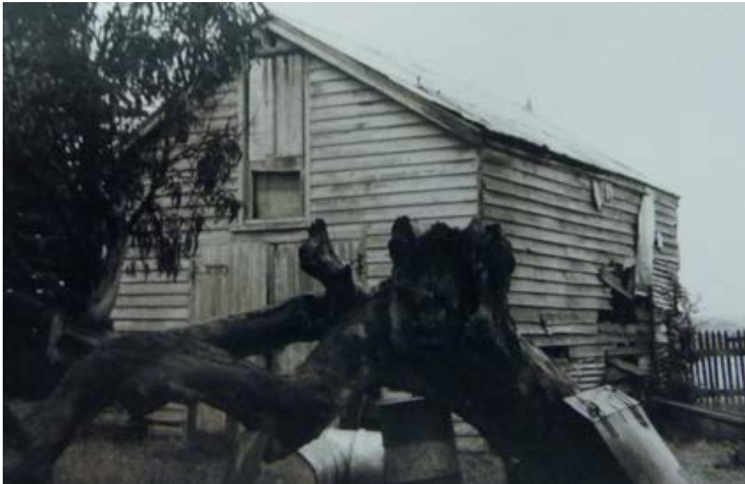
Figure 56 Amess stable looking south-west (undated, pre-1980)
