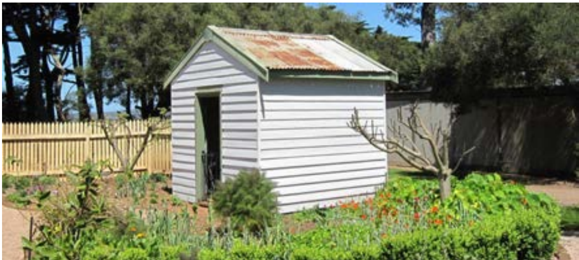
Figure 59 View of the wash house from the north-east
