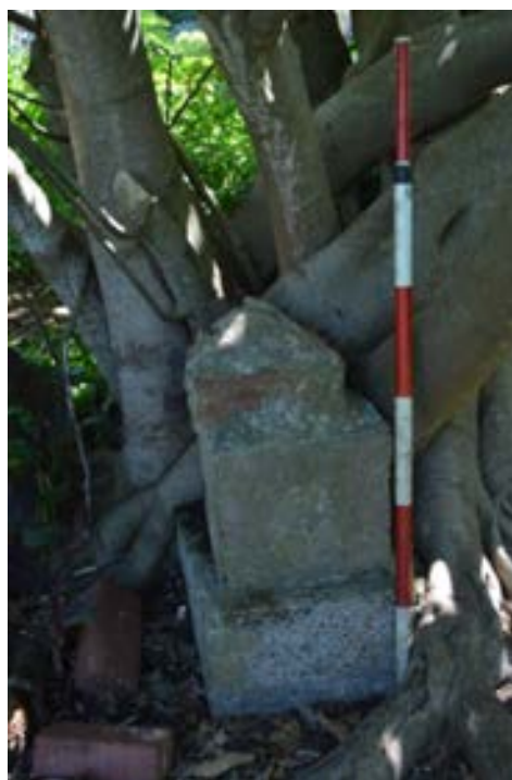
Plate 12: Concrete stumps for a tank stand in the garden.
