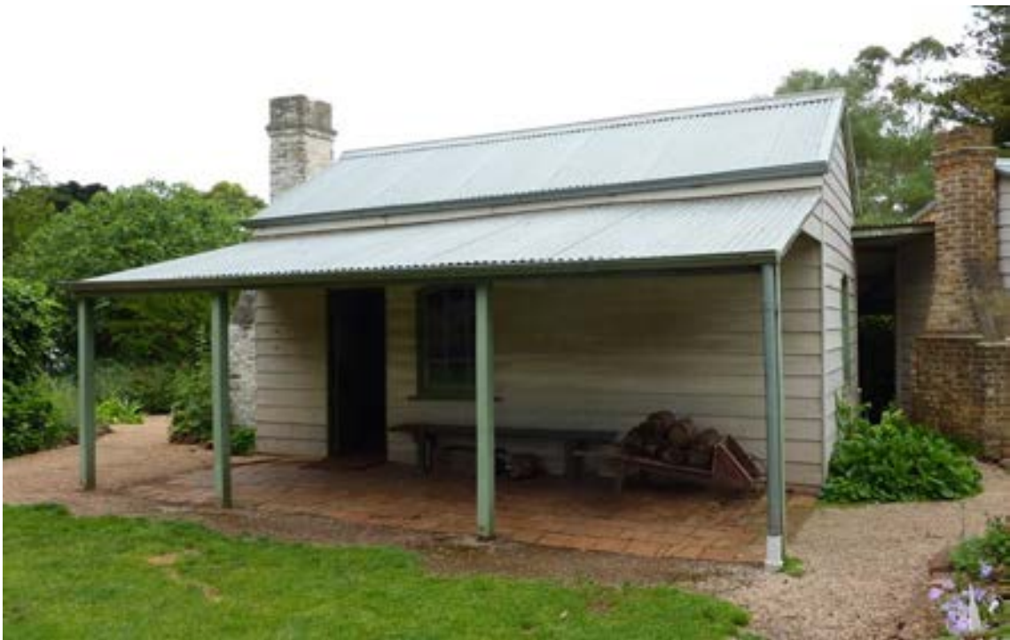
Figure 36 Kitchen cottage: west elevation
