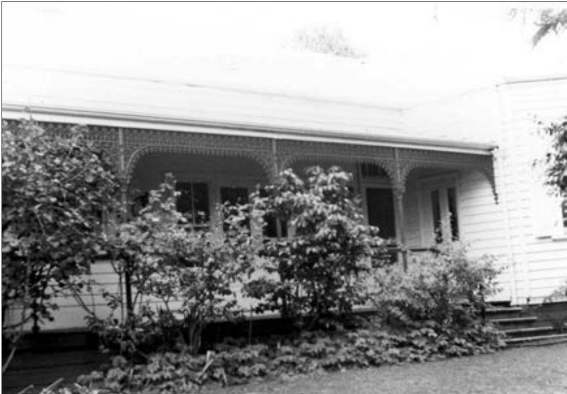
Figure 31 Amess house after completion of restoration work, 1984 Source: John Collins collection, State Library of Victoria
