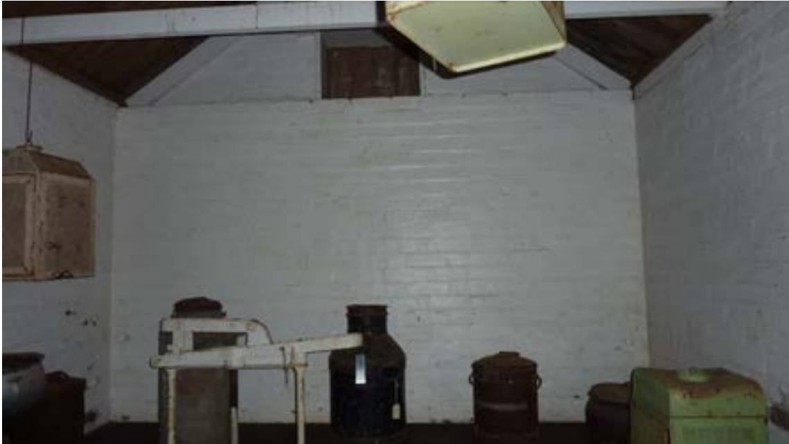
Figure 54 Amess cellar interior
