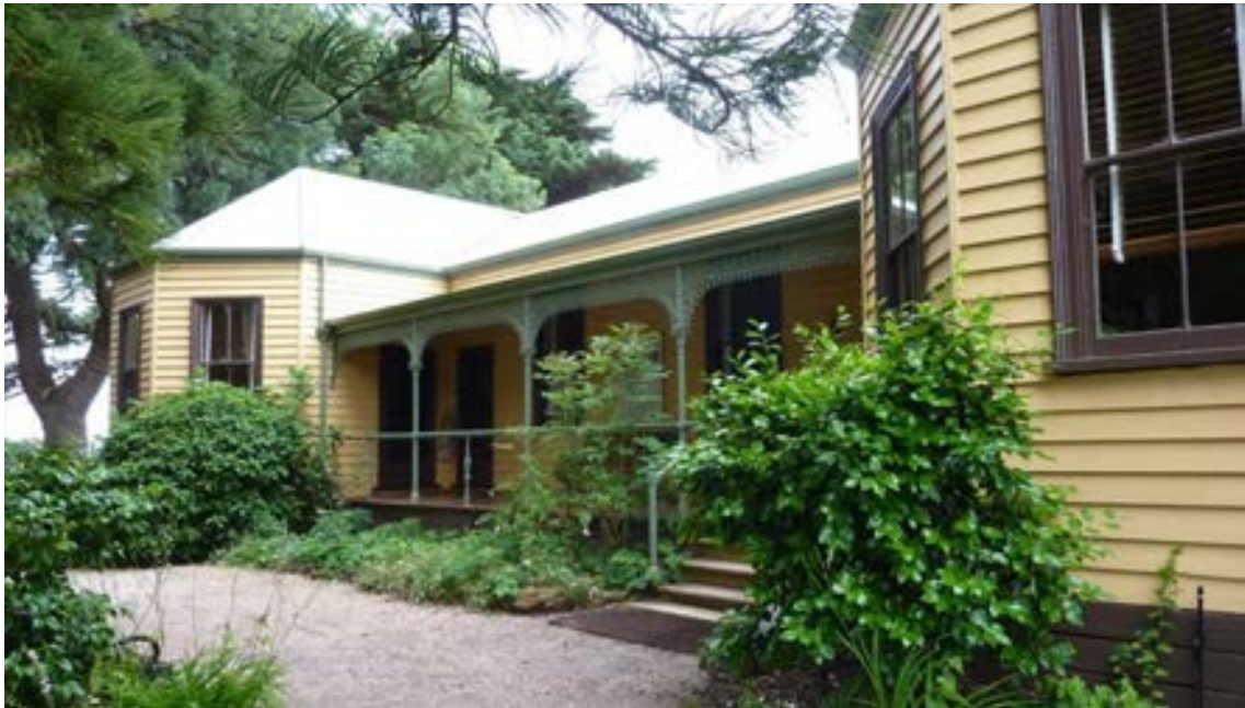
Figure 45 North-east facade of the Amess house
