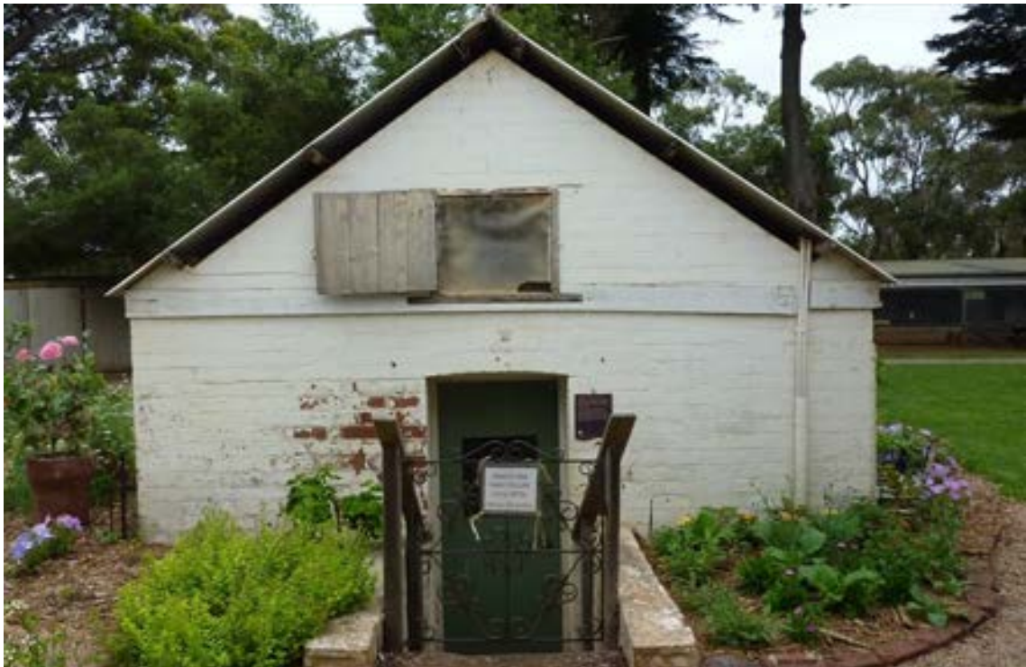
Figure 52 Amess cellar as viewed from the east
