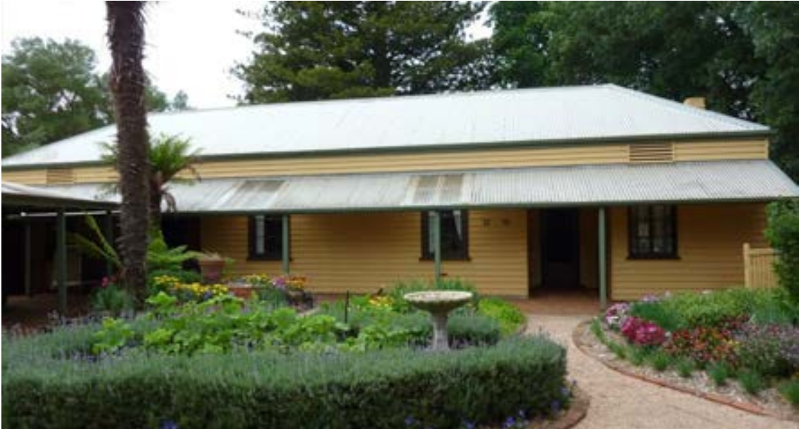
Figure 46 South-west elevation to the rear of the Amess house
