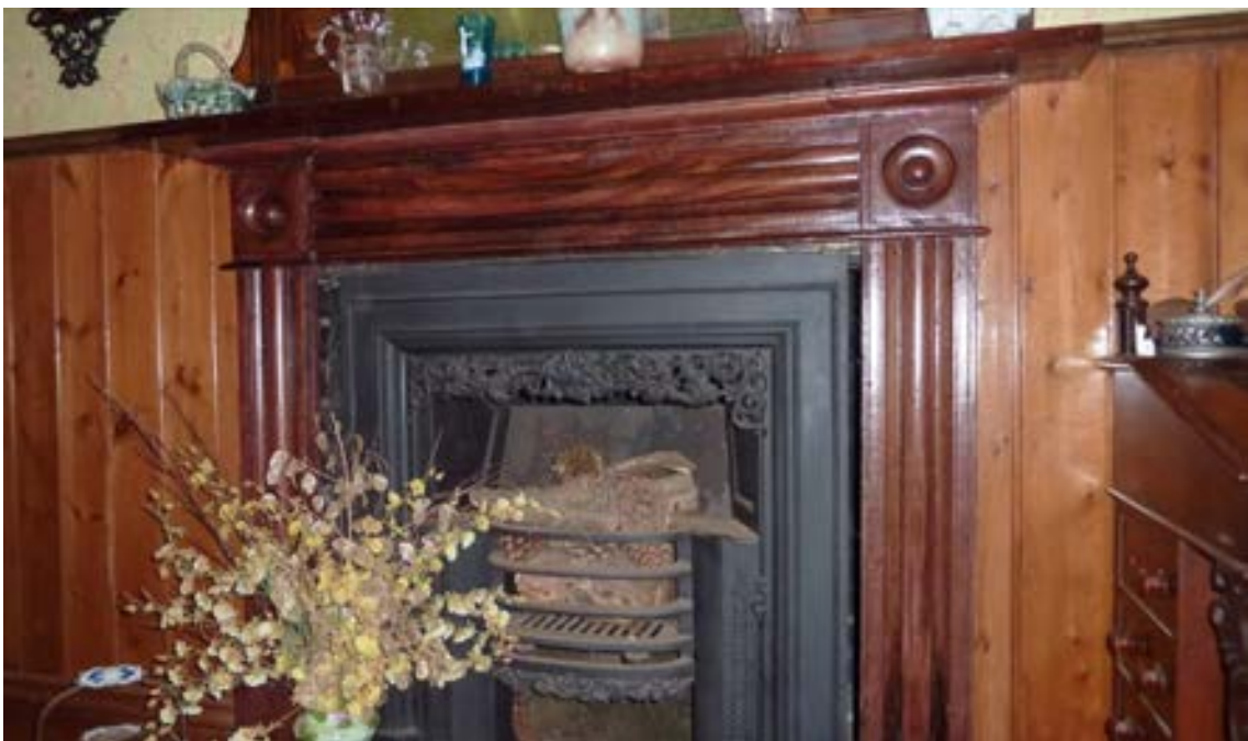
Figure 51 Amess house sitting room mantelpiece and fire surround detail
